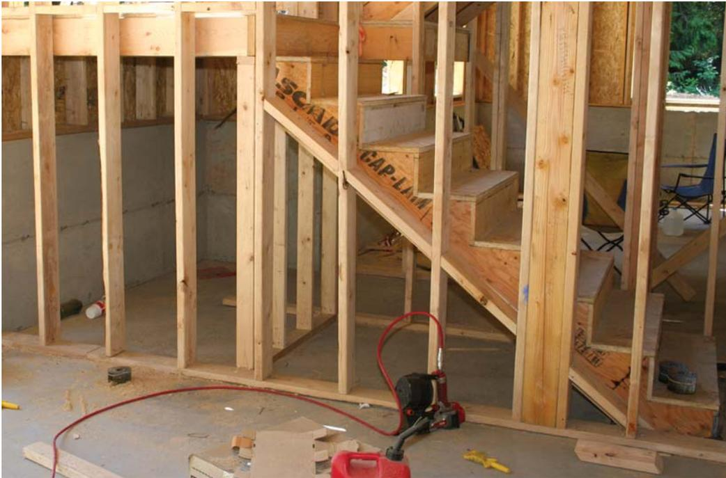
**Figure 2.** Sloped blocking beside the stringers and horizontal blocking at the landing separate the concealed space below the stairs from the stud bays above.
