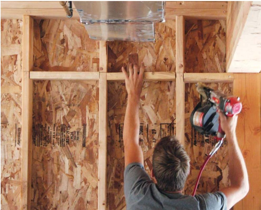
The purpose of fire blocking is to prevent fire from spreading through the concealed spaces of a building. It works by dividing framing cavities into separate compartments, slowing the passage of flames and combustion air.
