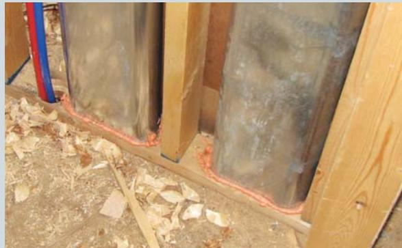
The red caulk around these pipes (top) is approved for use in fire-rated assemblies. The orange polyurethane spray foam around the ducts (above) is not intended for use in fire-rated assemblies, and may or may not be accepted by building officials for sealing penetrations through fire blocking.
