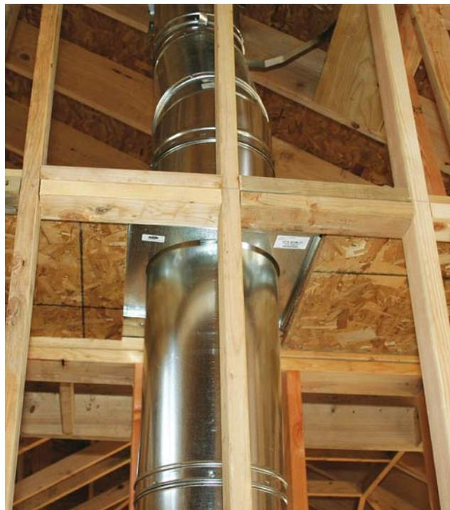
**Figure 3.** To separate the chimney chase from the attic, the author installs a 3/4-inch OSB fire block at the level of the ceiling. A metal fire stop fills the gap that is required between flue and OSB.
